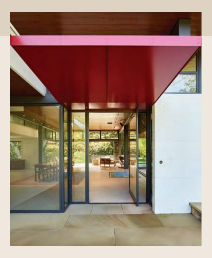
Hope's custom steel slide and fold windows and doors were selected to open a full-length back wall when desired. The narrow frames were designed to unlock and fold away from each other, achieving an open wall that includes two entirely open 90-degree corners. This cornerless feature plays an important role in allowing the house to be opened up and connected to the natural surroundings.
